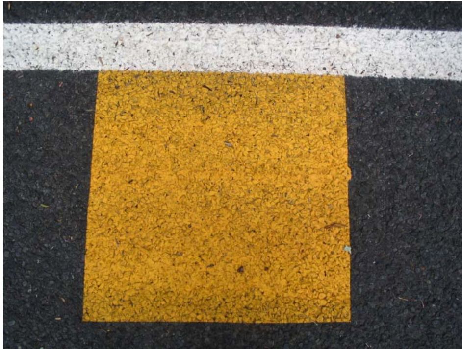
Figure 2.5 Pavement markings used for peripheral transverse lines treatments
