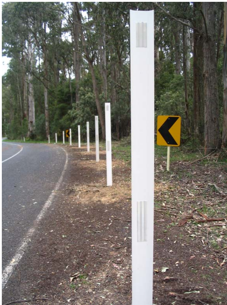
Figure 2.7 Treatment Site 2 - Curve Enhancement through Guideposts – Single Curve
