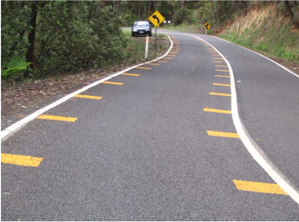
Figure 2.4 Treatment Site1 – Peripheral Transverse Lines – Single Curve
