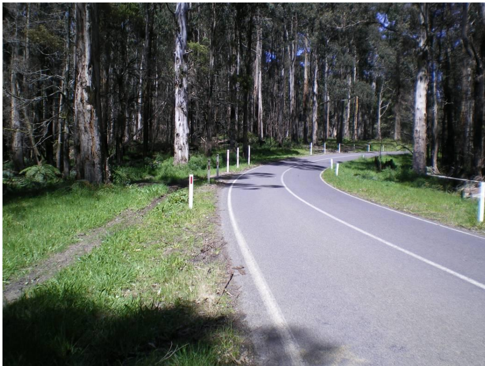
Figure 3.3: Site C – Treatment site
