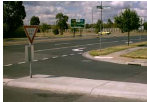
Fig 2. Use of splitter island and line marking to improve intersection delineation
