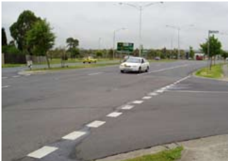
Fig 2. Use of splitter island and line marking to improve intersection delineation
