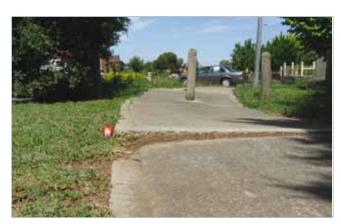
Figure 10: Slab misalignment
