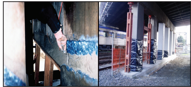
Fig 1: Trowel applied cementitious mortar (L), Cementitious mortars and grouts require curing in accordance with good concrete practice (R)
