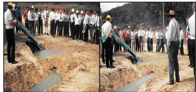
Fig. 1 Highly flowable fill discharged directly from chute, passing through restricted opening
