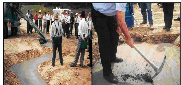
Fig. 2 Highly flowable fill travels over long distance to self level and self compact (L), Low strength flowable fill can be re-excavated using hand tools (R)
