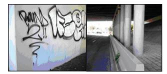
Fig. 1 Repeated painting out of graffiti, previous markings bleeding through (L), Long life anti-graffiti coating typically 3 m above ground level (R)
