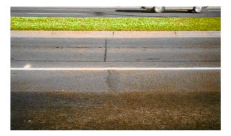
Tranverse cracking in "saw cut and seal" joints. Note the reflective cracking does not extend into the BSRA section (foreground).
