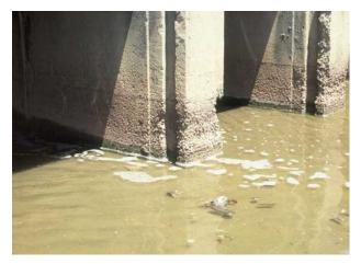
Figure 1: Concrete bridge pier damaged by acidic runoff from ASS.
