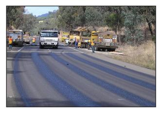
Photo 1 - Pre-sprayed road surface
