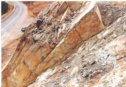
Figure 7: Weathering and adverse defect orientations.
