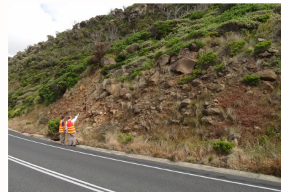
Figure 4: Loose rocks on batter face.
