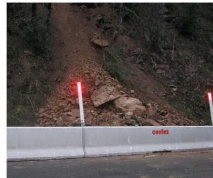
Figure 10: Temporary rockfall catch fence.
