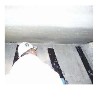
Fig. 2 Placement of the FRP with correct orientation and placement tolerances
