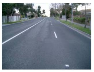
Figure 2 – Stripping of a spray seal applied to UTA.
