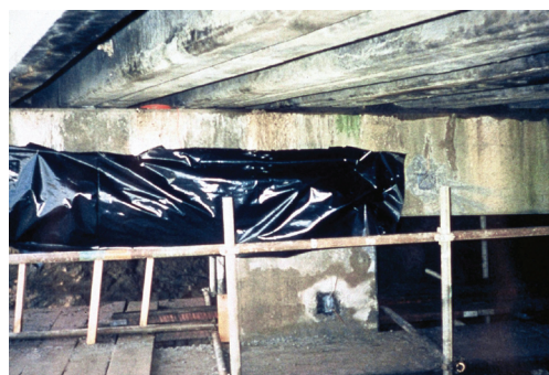
Figure 3: Curing of cementitious patch repair
