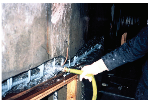
Figure 1: Surface preparation, saw cut and exposure of steel reinforcement and pre-wetting. Application of steel primer.
