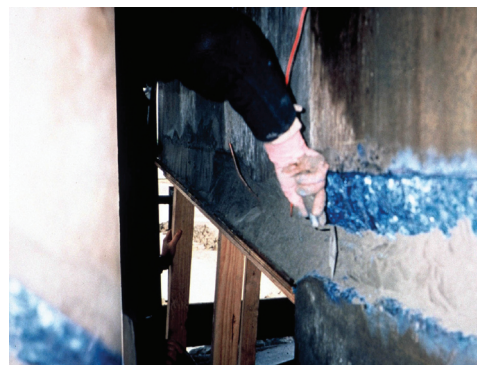
Figure 2: Substrate bonding coat and application of repair mortar.
