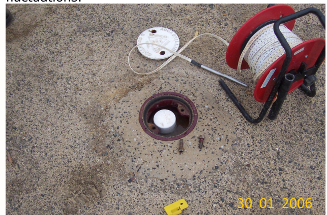
Figure 4: Standpipe and dip meter.
