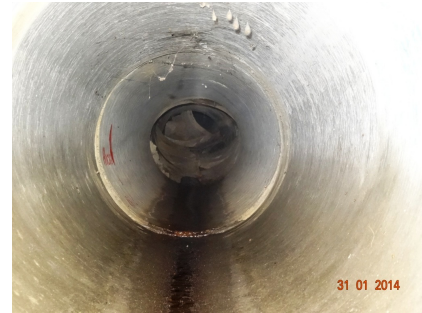
Figure 8: Leaking culvert.
