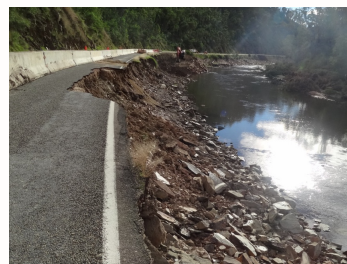
Figure 6: Erosion of river bank.
