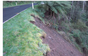
Figure 2: Slumping of soil.
