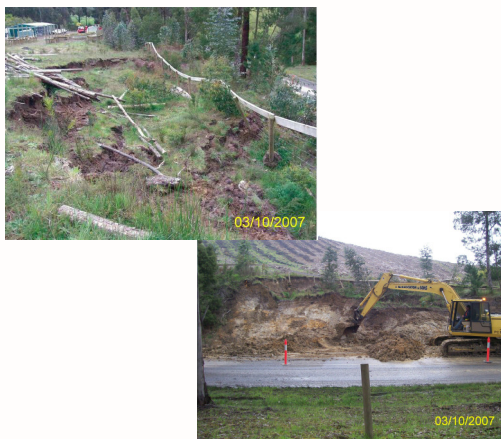
Figure 1: Rotational failure.
