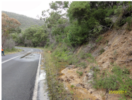
Figure 7: Blocked table drain.
