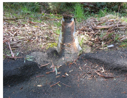
Figure 10: Asphalt bund discharging to flume on soil fill batter.
