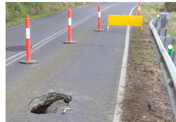
Figure 4: Cavity created by piping.
