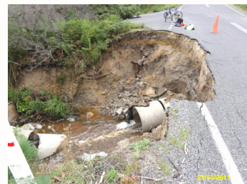
Figure 5: Erosion at culvert outlet.
