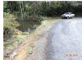
Figure 3: Embankment fill acting as a dam.
