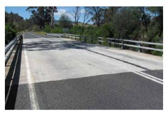
Figure 1: Concrete wearing surface
