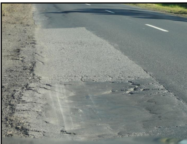
Figure 6. Significant failed area with loose pieces of pavement.
