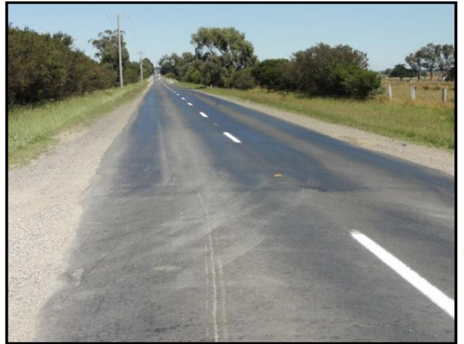
Figure 8. Significant flushed wheel paths in a 100kph zone.
