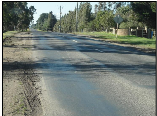
Figure 3. Significant shape loss.
