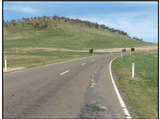
Figure 1. Significant number of potholes.
