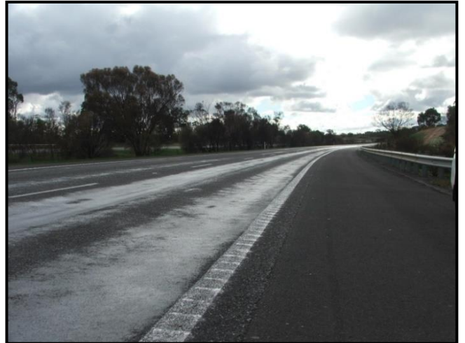
Figure 7. Significant flushed wheelpaths in a 100kph zone.
