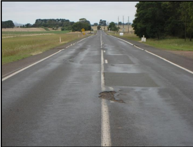
Figure 4. Significant failed patches with shape loss.
