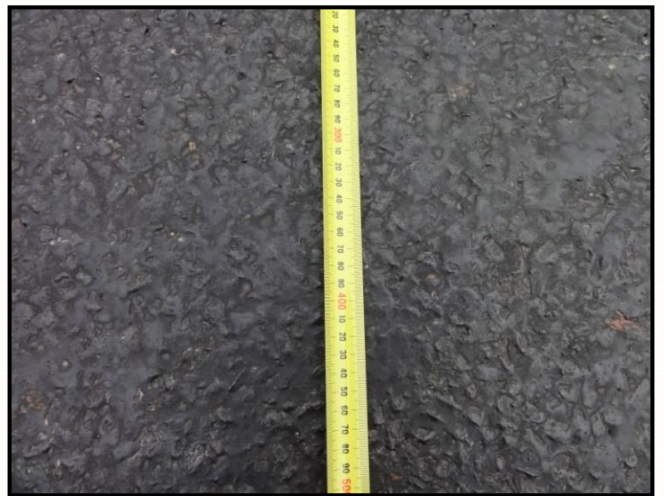
Figure 9. Close-up of flushed surface.
