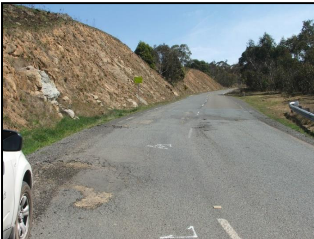
Figure 5. Significant failed areas with shape loss and loose pieces of pavement.
