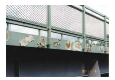
Figure 7.1: Surface preparation which is below the minumum required, or the omission of primer of intermediate coating, or coatings which are below the thickness specified, may lead to premature failure of the coating system.
