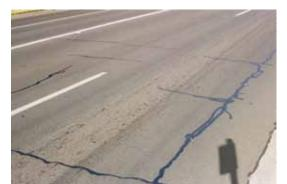
Rating 1 Extent: Minor Comments Single cracks in asphalt
