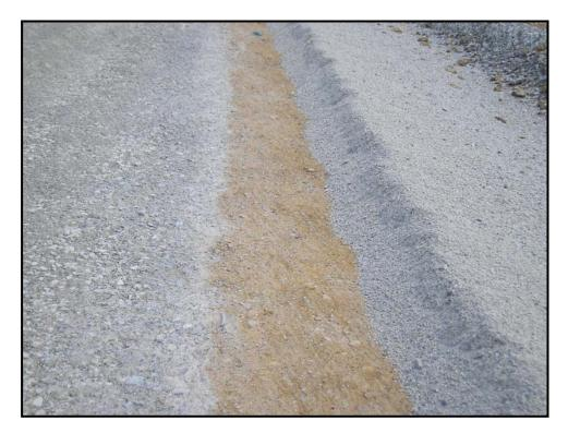
Figure 3 : Excess Material Swept from Compacted Layer
