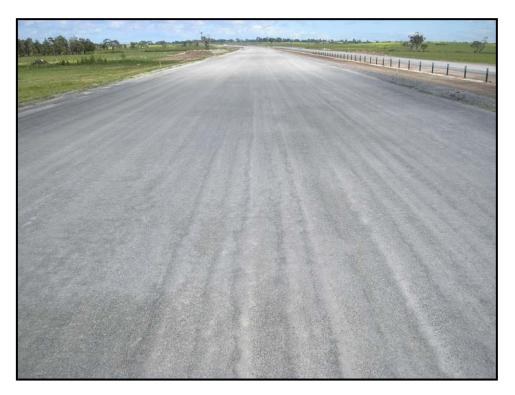
Figure 8 : Excessive Slurrying of Fines
