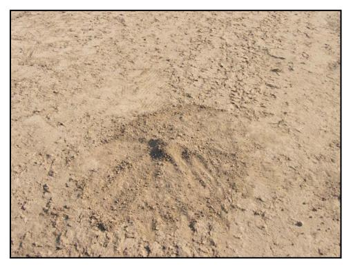
Figure 2 : Layer of Fine Material on Top of Crushed Rock
