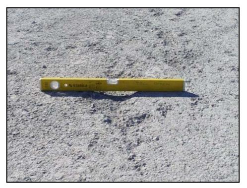
Figure 5 : Tearing of Pavement - Ravelling
