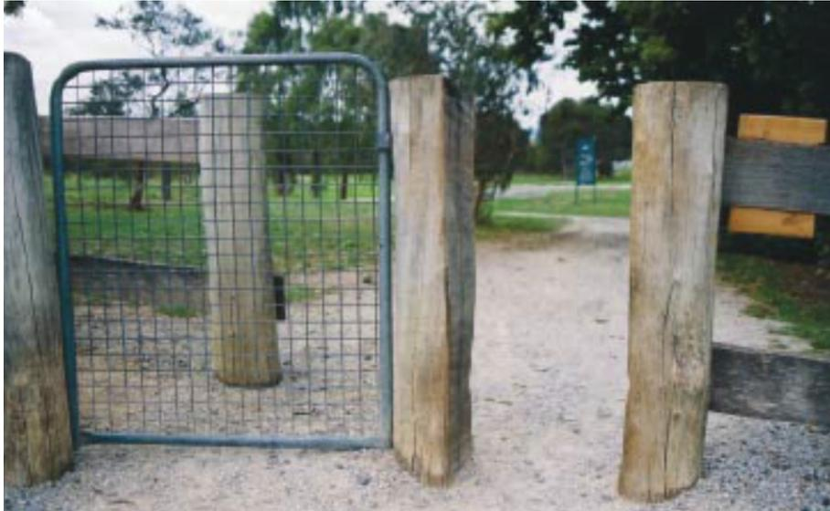
**Figure 7: Terminal treatment with an opening that cyclists find difficult to pass through**
