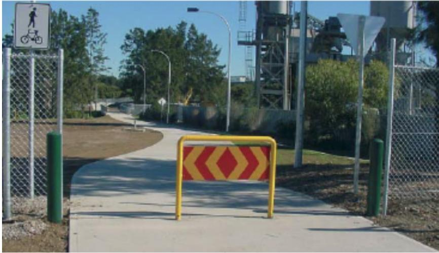
**Figure 12: Example of preferred ‘U’ – Rail and target board to prevent motor vehicle access (courtesy RMS, NSW)**
