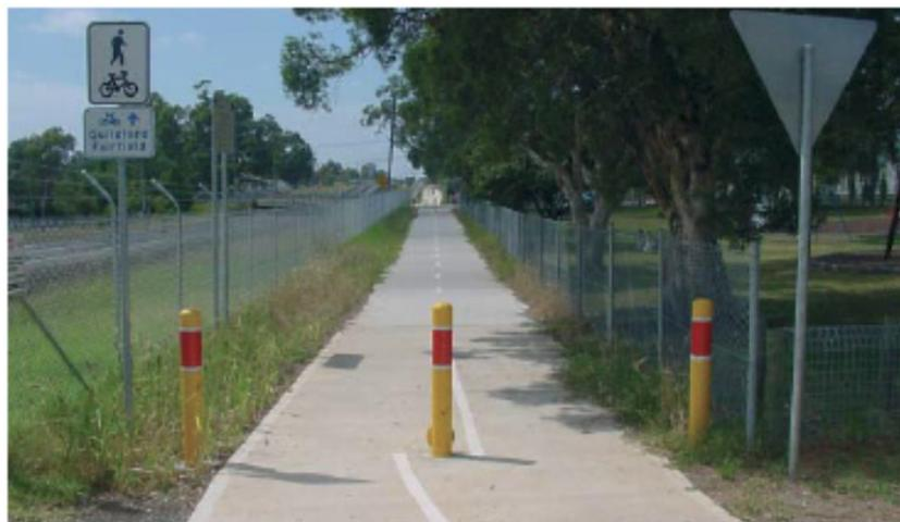
**Figure 11: Example of preferred bollard treatment to prevent motor vehicle access (courtesy RMS, NSW)**
