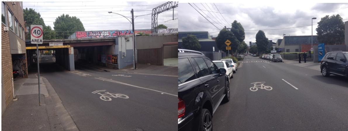
The above photos shows 'sharrows' being used to compliment traffic management treatment that support low speed environments.
