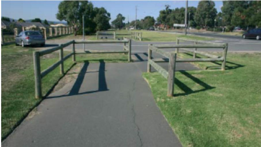
**Figure 9: Offset bicycle path on Kelletts Road, Rowville**
