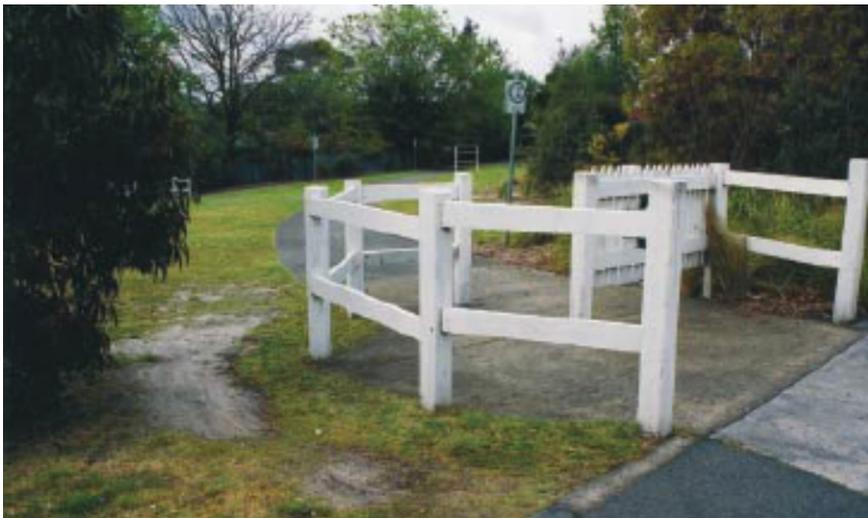
**Figure 6: Terminal treatment that cyclists avoid by cycling to the left**
