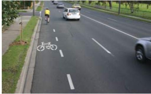
**Figure 2: Marking details of wide left lane**
